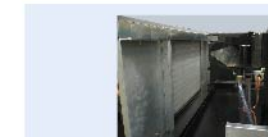
DX-coil (Direct expansion coil)
